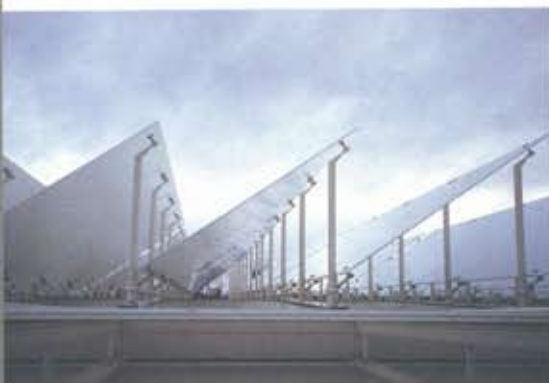
8. Brises soleil, looking west.
