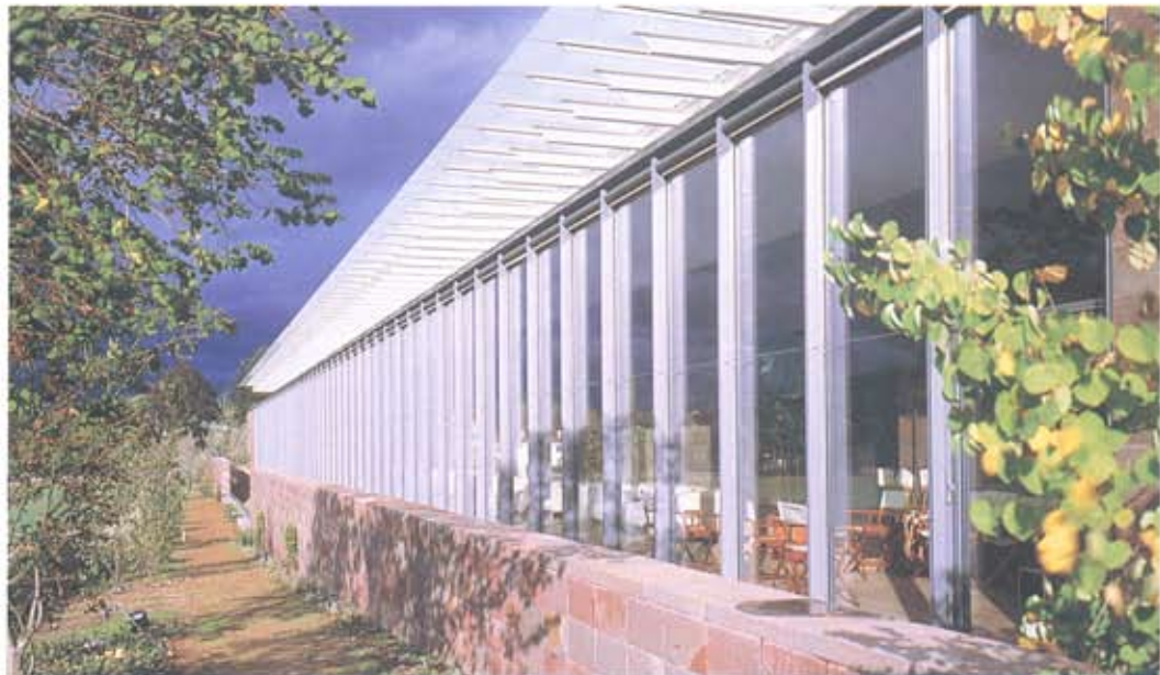
6. The west wall, looking north.
